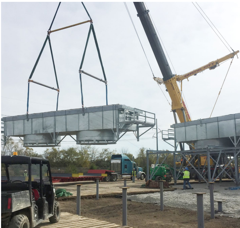
Cooler being installed at Chandlersville
